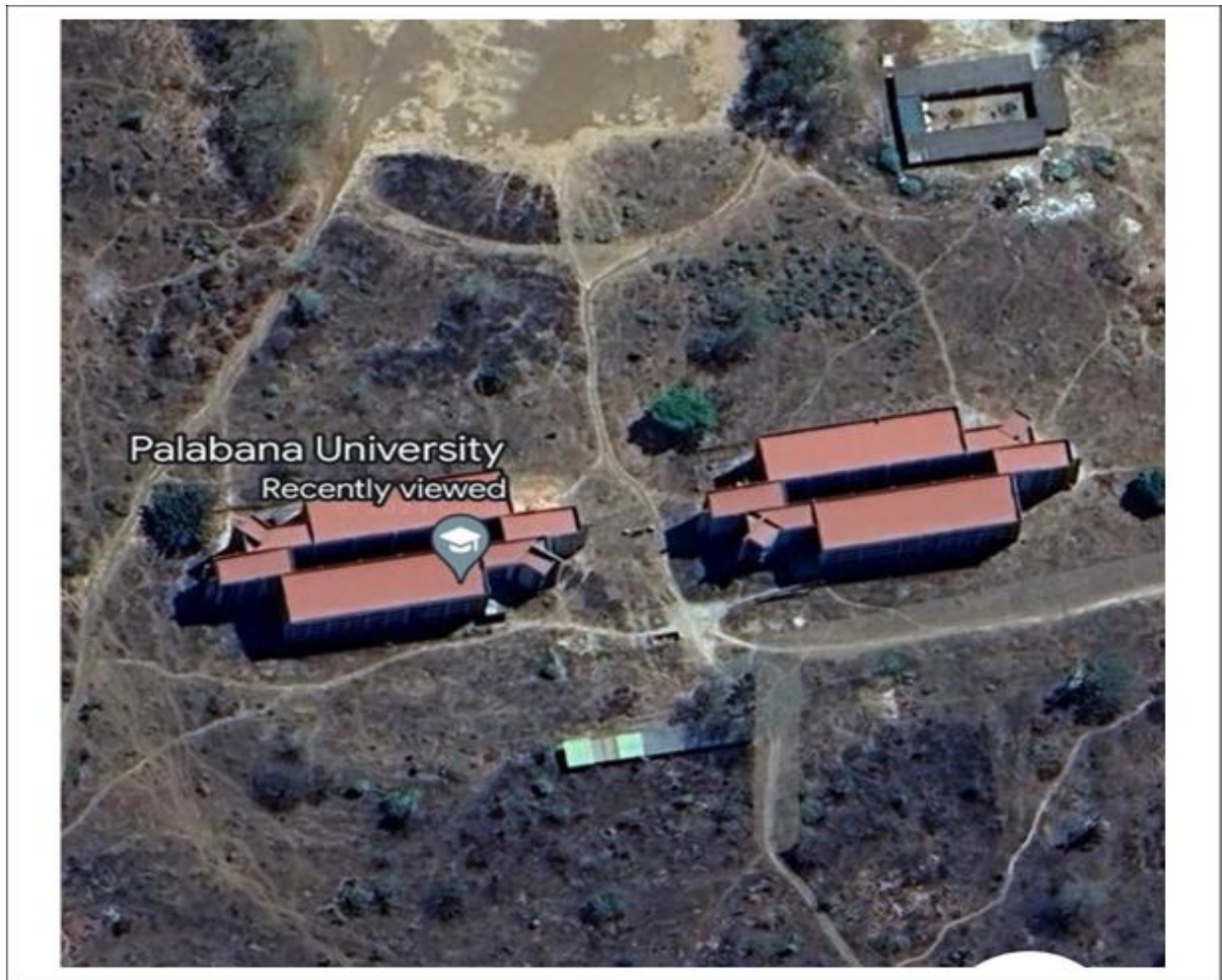
Aerial view of the two uncompleted student hostels (The roof tops are being targeted for placement of solar panels).
