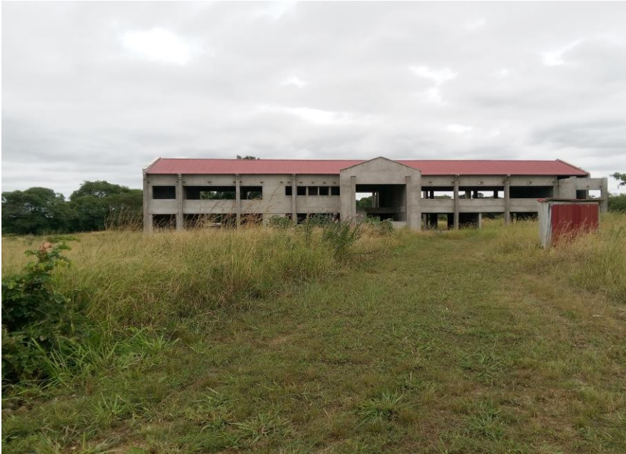
A building housing Lecture rooms that needs urgent attention for completion.
