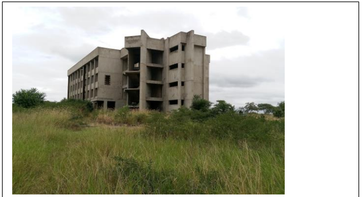
One of the uncompleted Student Hostel, observed from a Distance
